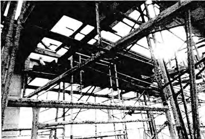
Gambar 3.11.7 Bekisting balok
