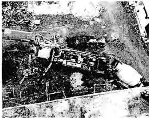
Gambar 3.8 mobile pump concrete
