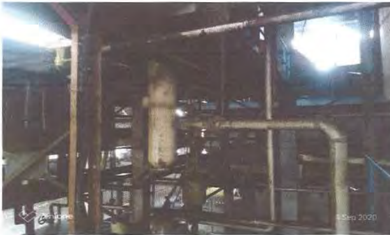
Gambar 3.7 Sand Cyclone
