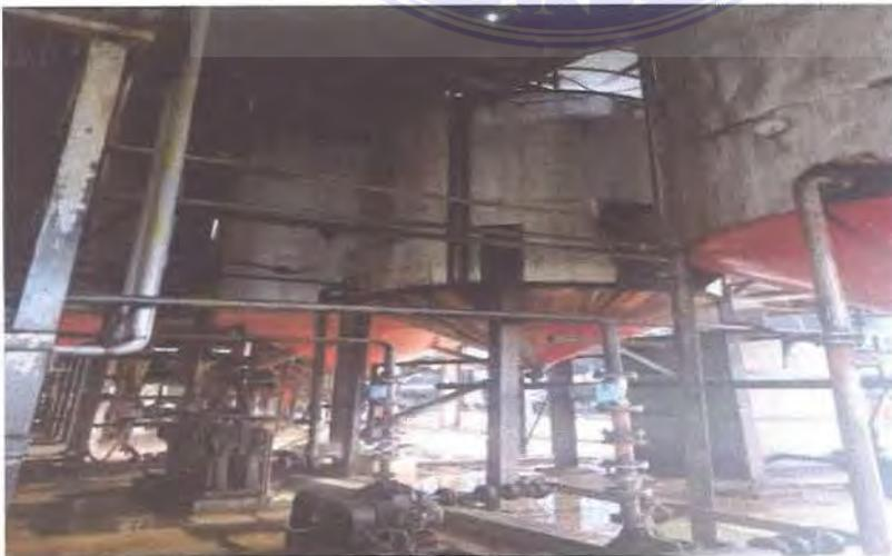
**Gambar 3.14 Vertical Clarifier Tank**
