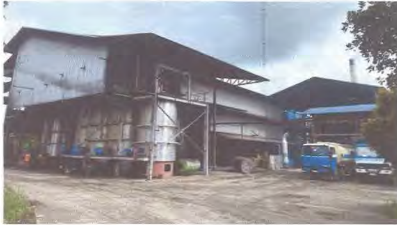
Gambar 2.1. Pabrik Kelapa Sawit PT. Mulia Tani Jaya
