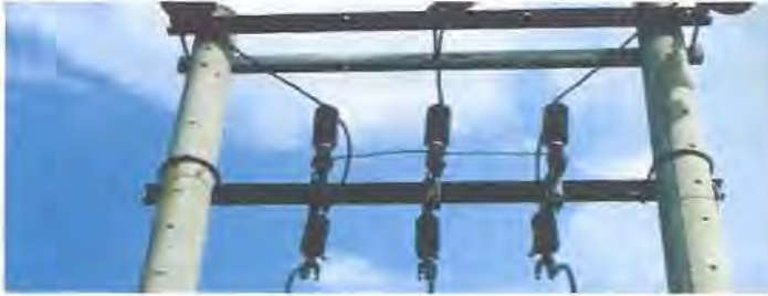
Gambar 2 14 Lightning Arrester
