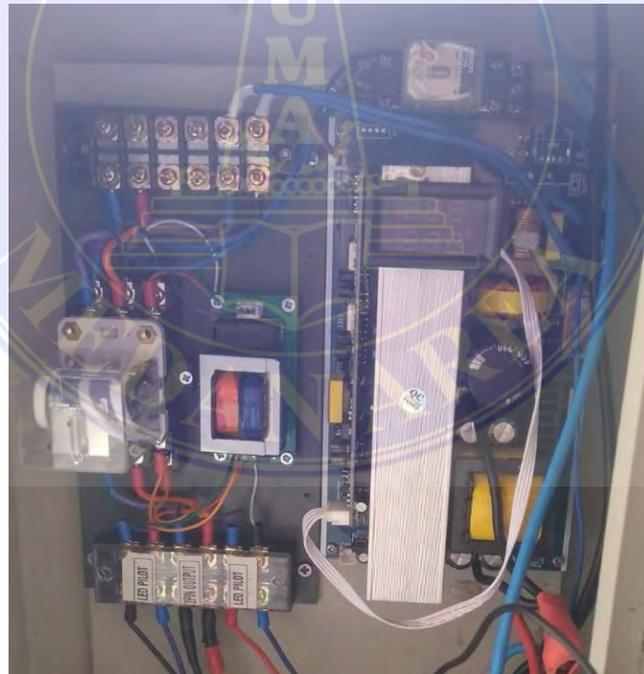
Gambar 2.7 : *Automatic Transfer Switch System (Sistem ATS)*
