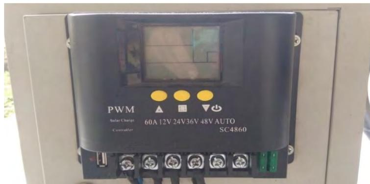
Gambar 2.5 : *Solar Charger Control (SCC)*
