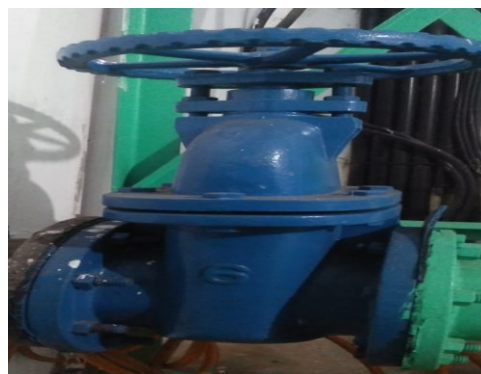
Gambar 3.4. Flange Gate Valve
