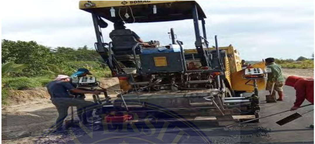
Gambar 2.2 *Asphalt Finisher*
