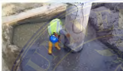
Gambar 2.3 Pemasangan Drop in anchor
