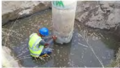
Gambar 2.1 Penandaan/marking posisi sensor (1,2 m)
