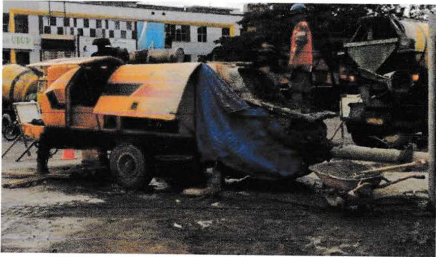
Gambar 3.1. Pump Mini Beton
