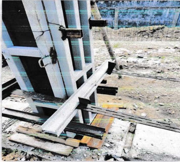
**Gambar 4.22** Bekisting Kayu Kolom
