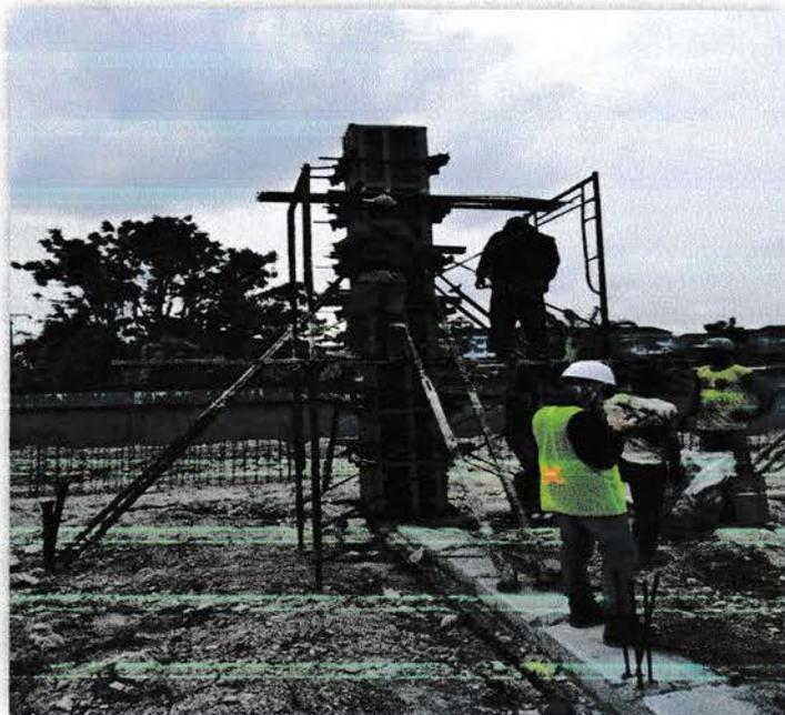
**Gambar 4.21** Bekisting Plat Kolom
