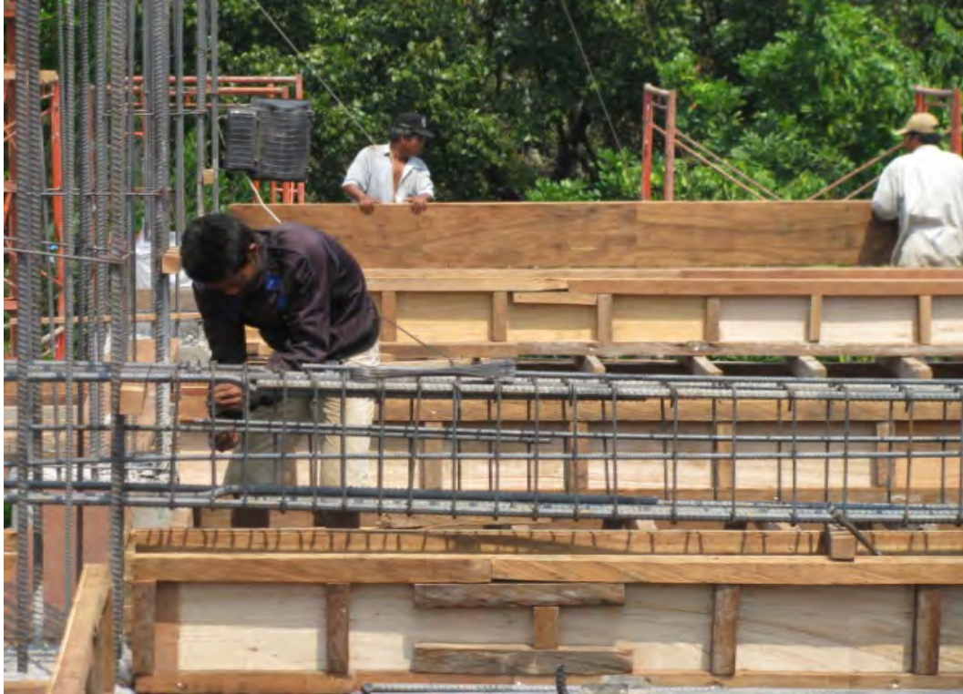
Gambar 3.2. Bekisting balok
