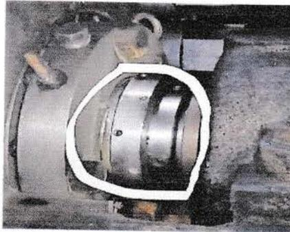
**Gambar 3.11** Mechanical seal pompa
