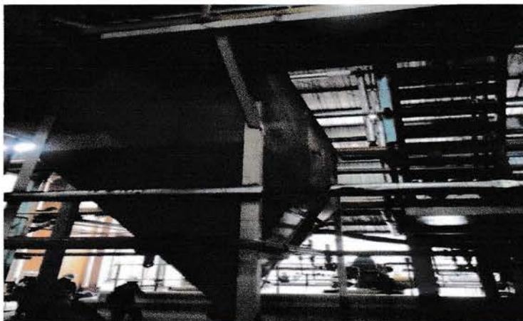
Gambar 3.9 *Sand Trap Tank*
