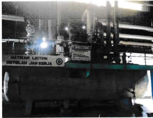
**Gambar 3.20. Back Pressure Vessel**
