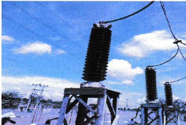
Gambar 2.16 Current Transformer (trafo arus)
