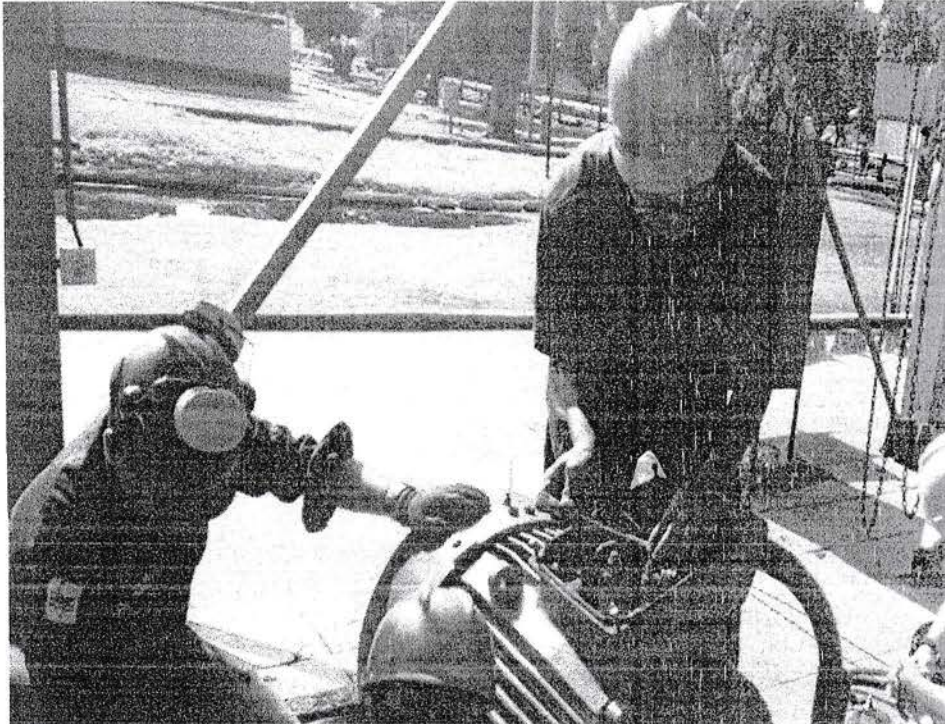
Gambar 3.4: Buka Cover terminal motor 380 V
