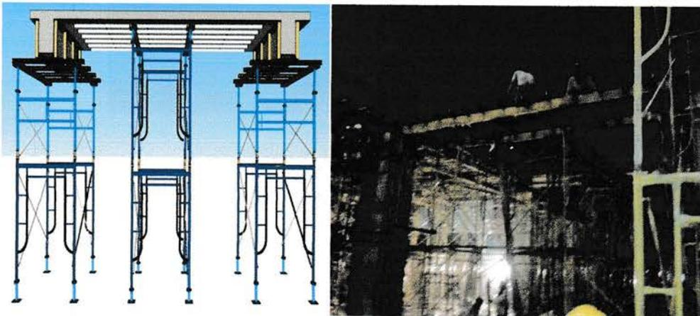
**Gambar 3.2. Bekisting balok**
