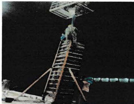
**Gambar 3.1. Bekisting kolom (bekisting dinding peri)**
