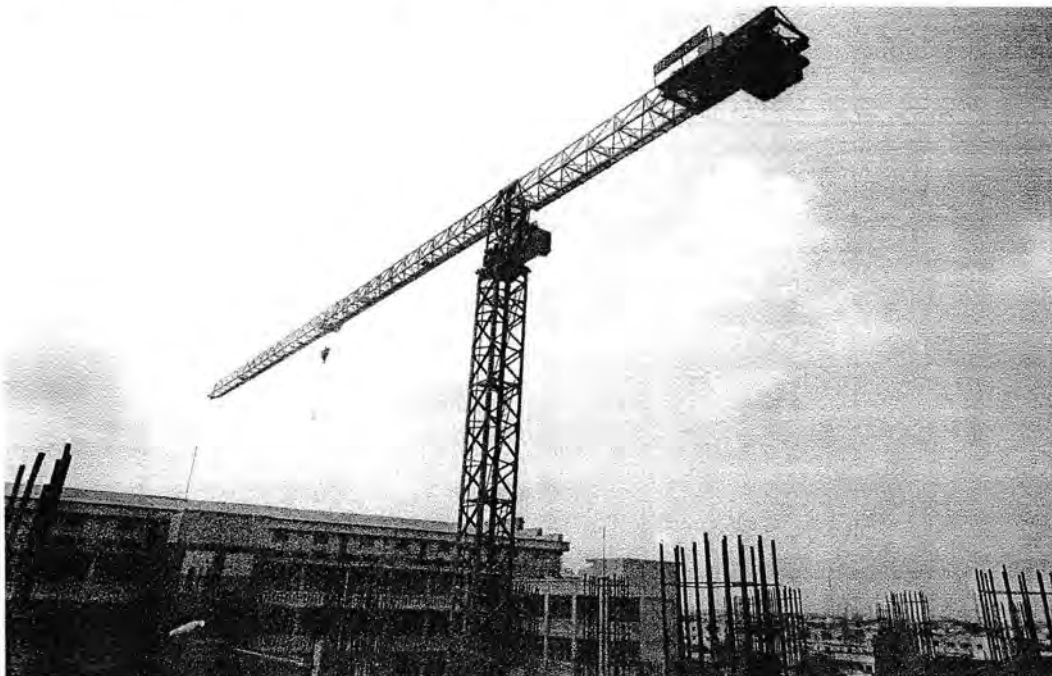
UNIVERSITAS MEDAN AREA Gambar 2.10.5 Tower Crane
