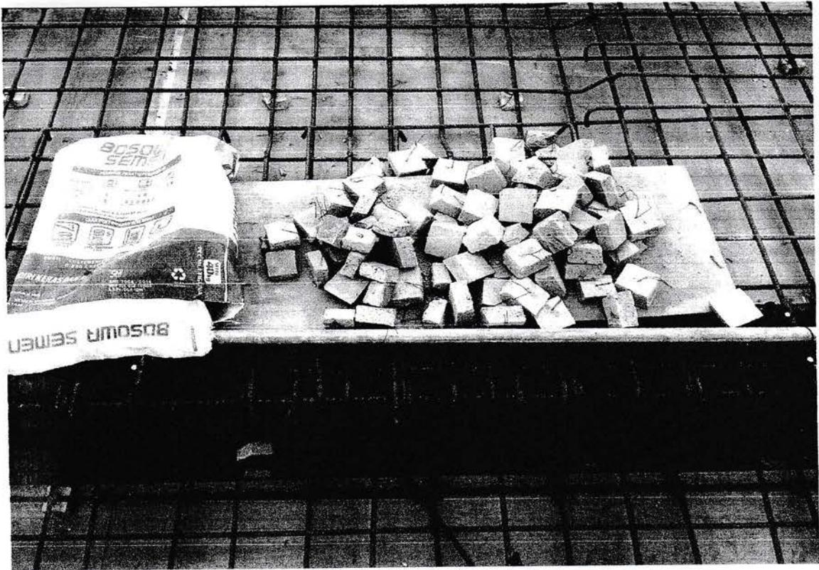
**Gambar 1.13 : Tahu Beton/Beton Decking**
