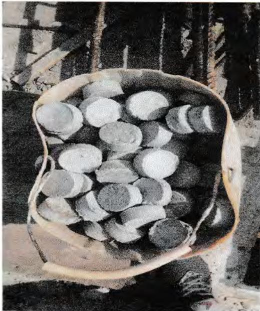
Gambar : Beton Daking
