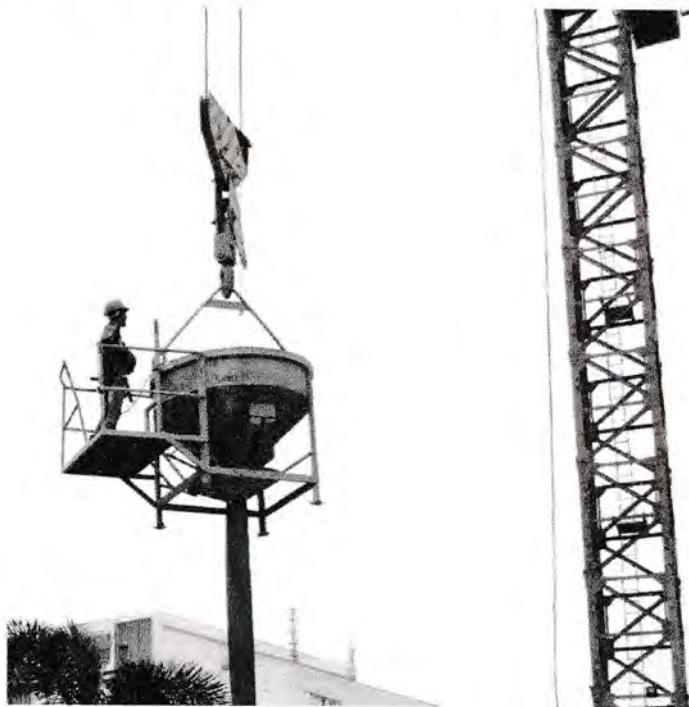
**Gambar 3.7 Concrete Bucket dan Pipa Tremie**
