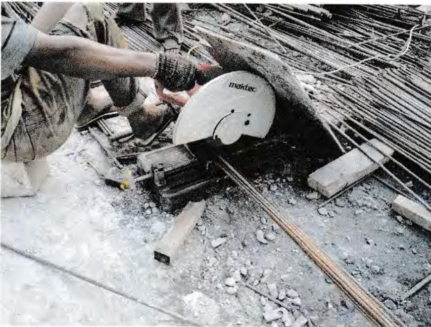
Gambar 3.16 Bar Cutter (Pemotong Tulangan)
