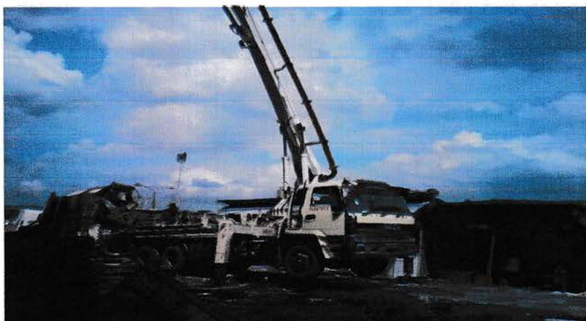
Gambar Pump Concrete
