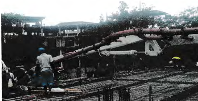
Gambar Pump Concrete
